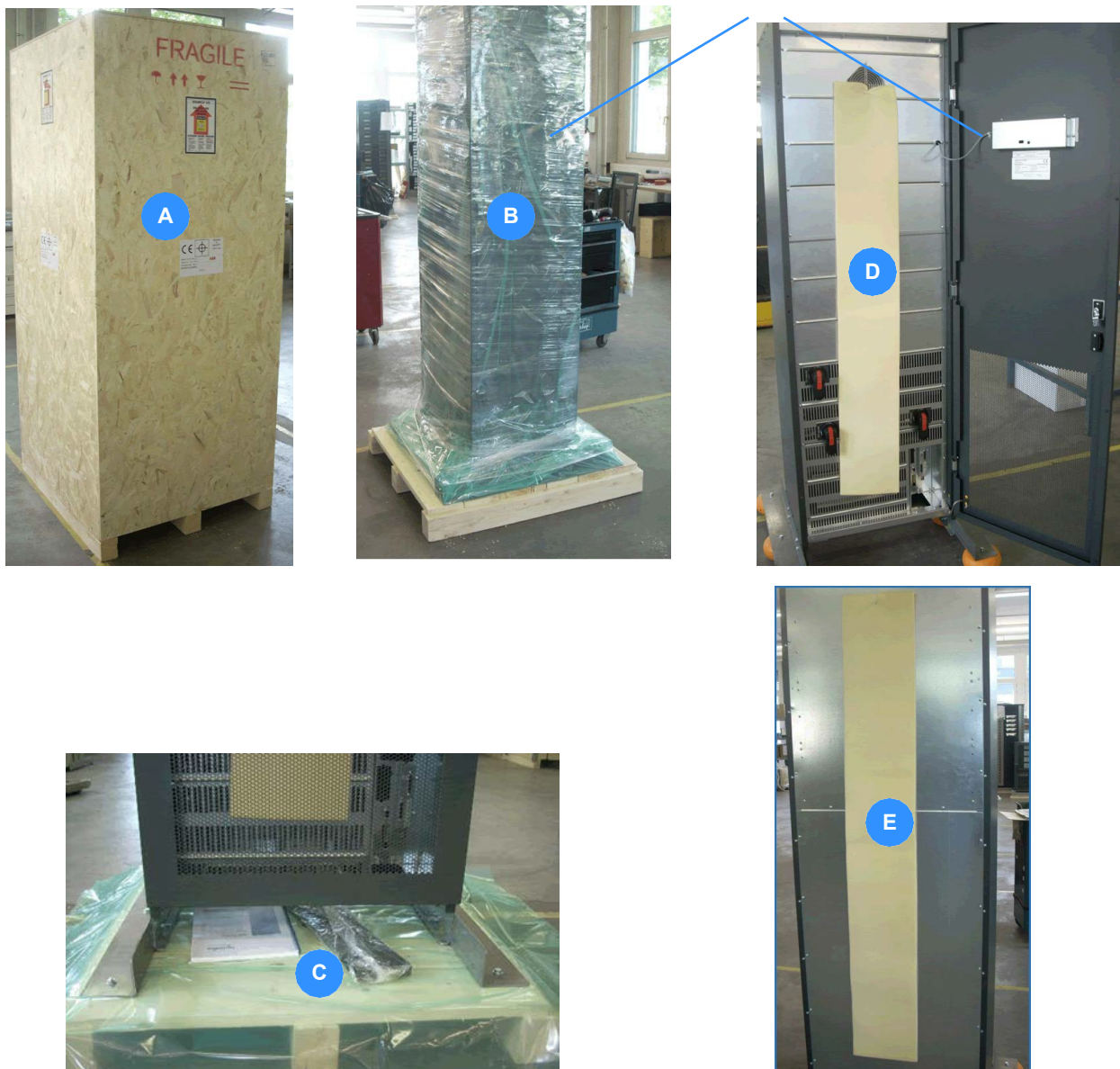
Figure 4.3 Unpacking the UPS cabinet (sea freight packaging)
